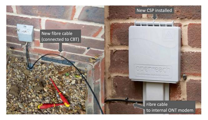
Normally the modem would be fitted on the inside of the wall at a suitable place normally next to your existing Master Socket, but it can actually be anywhere on an outside wall
